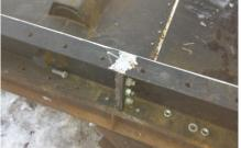
5. You can weld the flanged part together ore use sealing, depends on the deviation.
